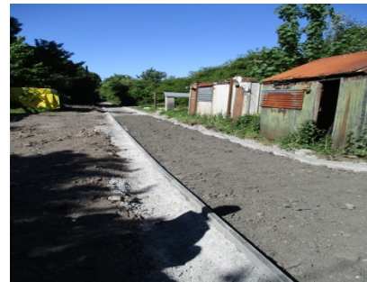
6 Core Path upgrade works at Dalintart
