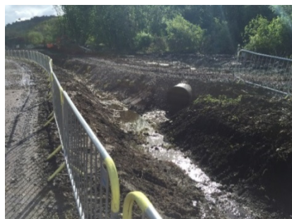
8a Culvert realignment works
