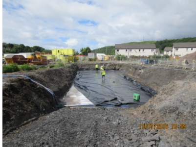
17 Preparation of site for attenuation tank
