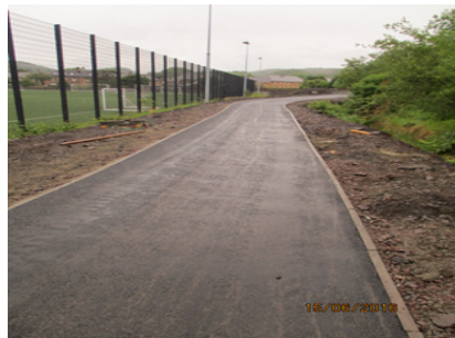
7a Completed Core Path adjacent to 3G pitch
