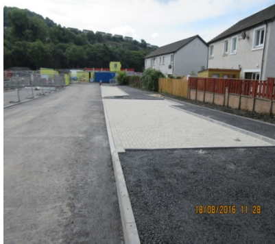
20a New access road and footpath to the rear of McCall Terrace
