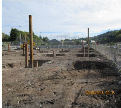
19a Piling installation
