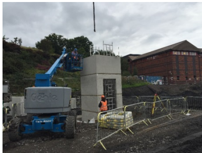
21 First lift shaft being constructed
