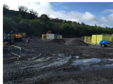
2 Preparation of site compound area
