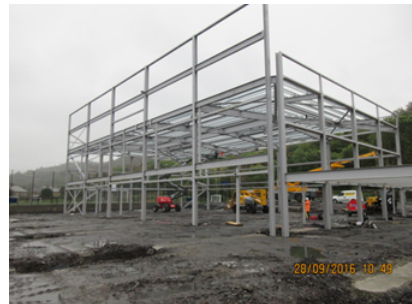
22 First sections of steelwork being erected
