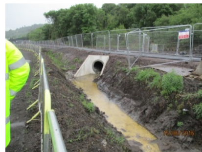
8b. Realigned culvert
