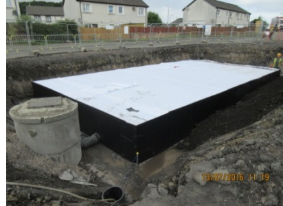
18 Attenuation tank installed
