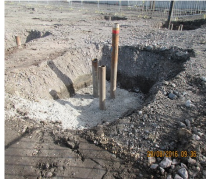
19b Concrete binding laid to enable piles to be cut to correct length
